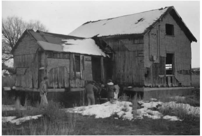
The Gully house undergoes repairs in 1981. Photo Credit Virginia Steele
