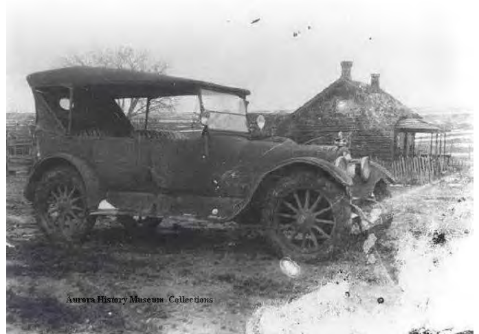
The Gully home in its original location near Mississippi and Chambers. Photo Credit: Aurora History Museum
